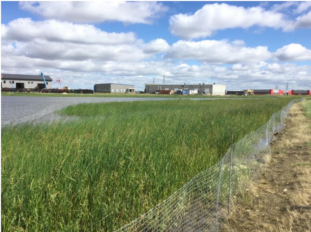
Figure 9. Emergent vegetation in a naturalized retrofit of a conventional stormwater pond in Winnipeg during the first year of vegetation establishment.
